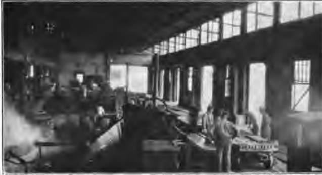
A. COOLING AND LOADING INGOTS, MICHIGAN SMELTER.
